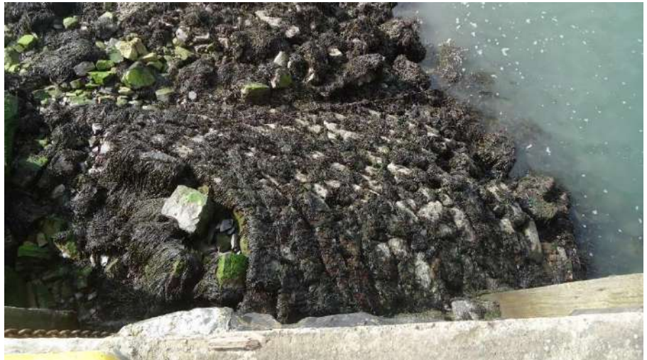
View looking down from quayside at the embrasure feature built in front of the stone quay at its southern end, to act as an armoured protection.
