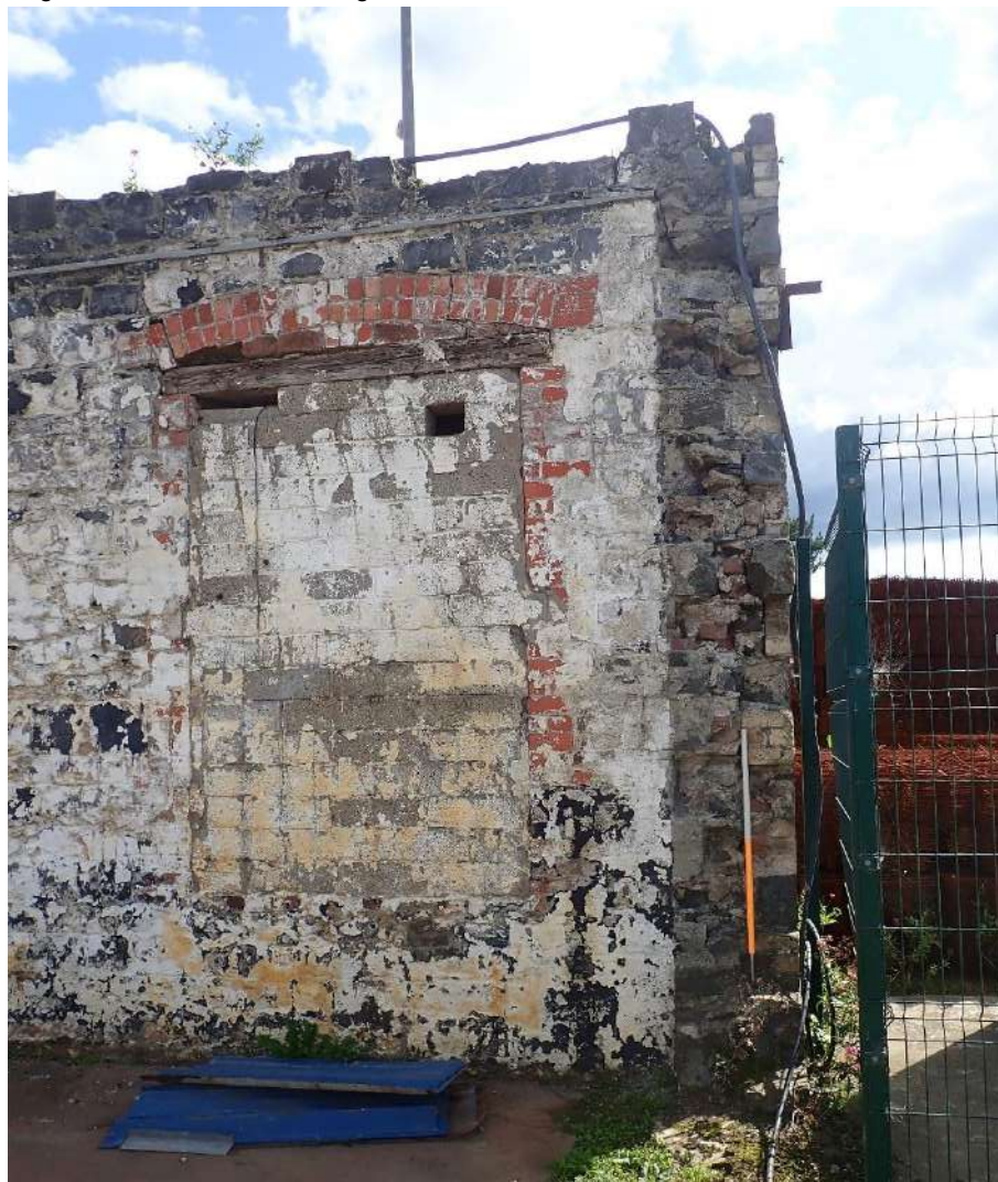
Engine Shed wall, west end showing wall end-wall fracture, view from north.
